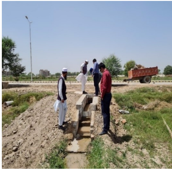
Inspection of flow meter structure
