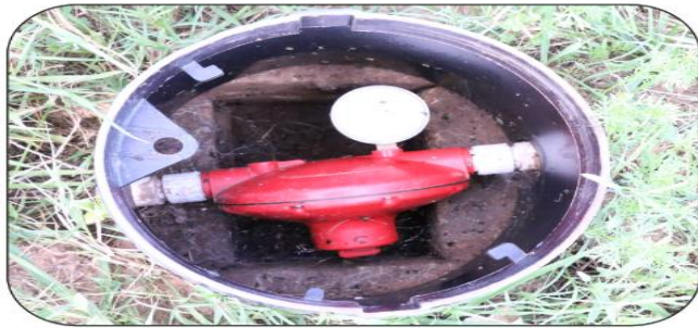
Adjustable Pressure Regulator (APR) and Pressure Gauge
