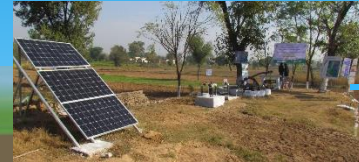
Solar Pump on Dug-well
