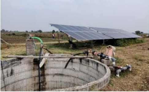
Figure 1- Solar irrigation setup in Botad district with farmer's dug well and solar panels.
