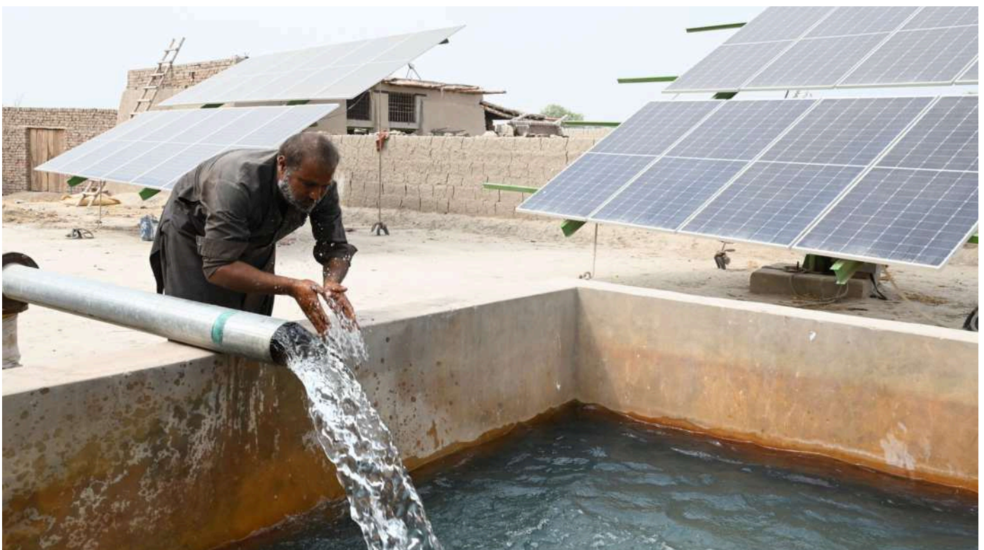
A farmer using the Solar tube well at Rahim Yar Khan, Punjab Province (photo: Amjad Jamal/IWMI).
