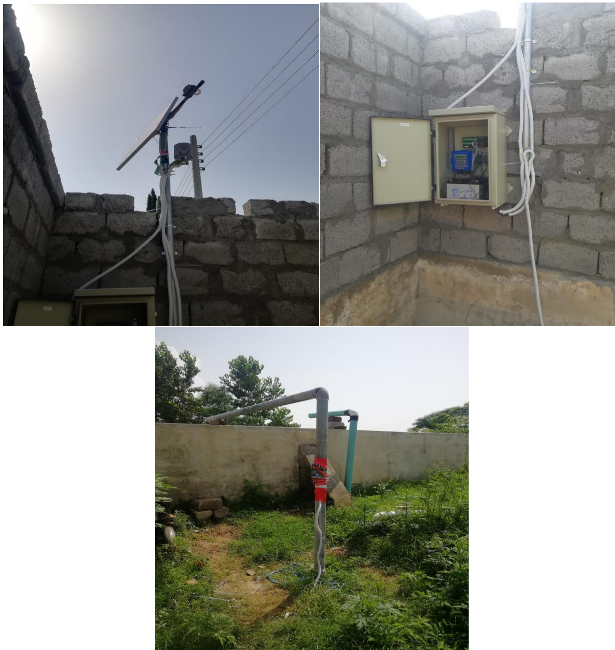
Site 1 – Solar Pump – Talagang
