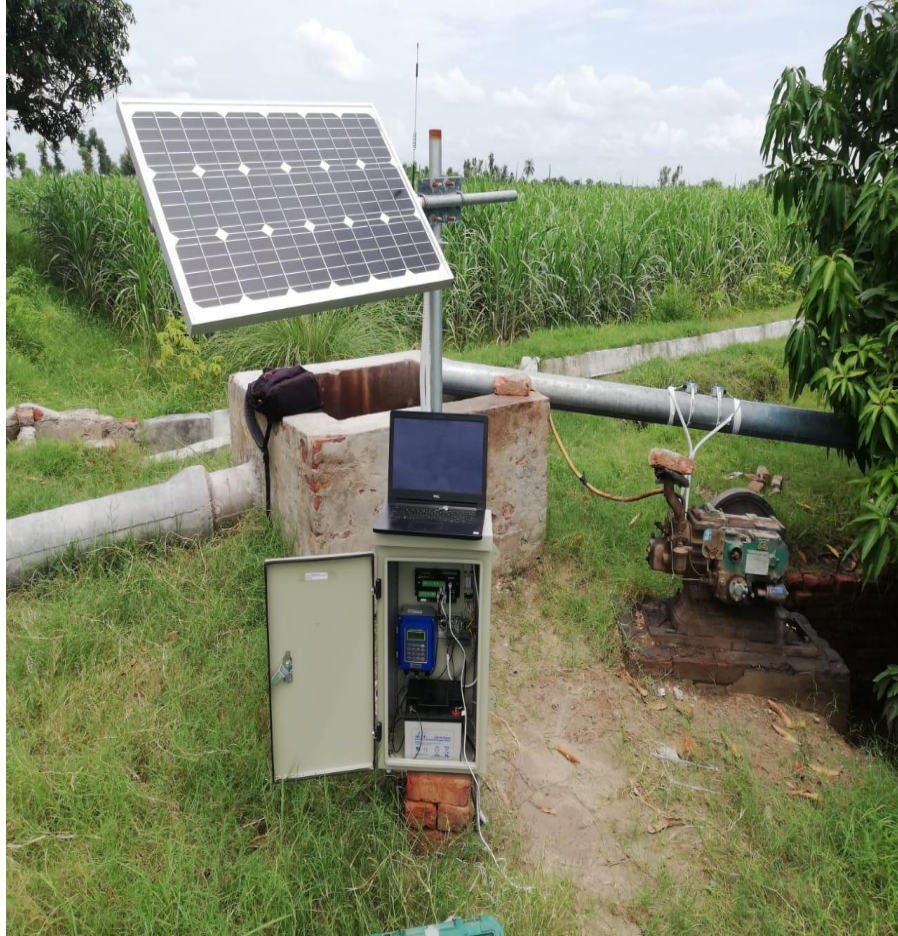
Site 12 – Diesel Pump - Khanpur
