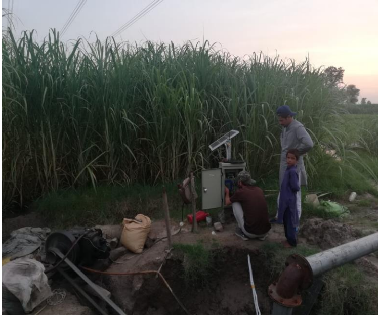
Site 7 – Diesel Pump – 18 Hazari
