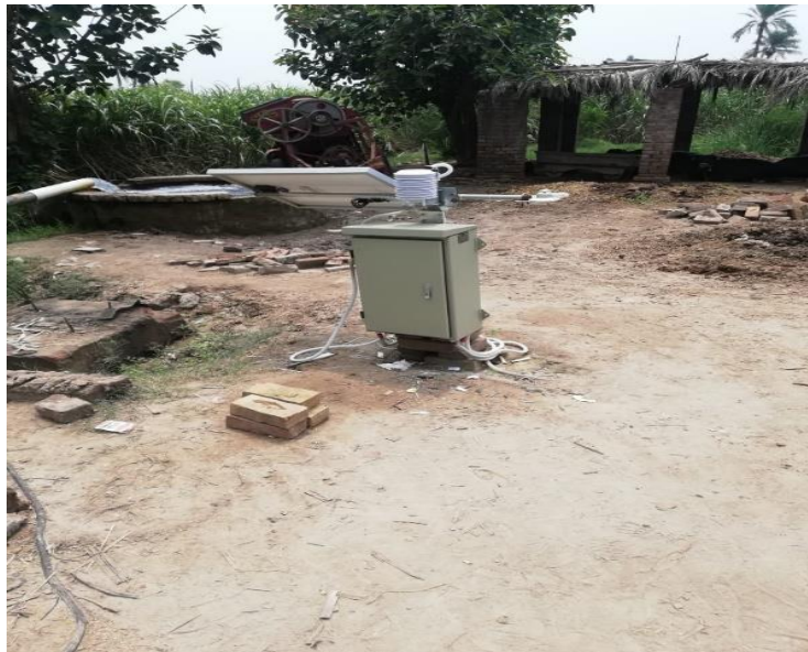
Site 8 – Solar pump – 18 Hazari
