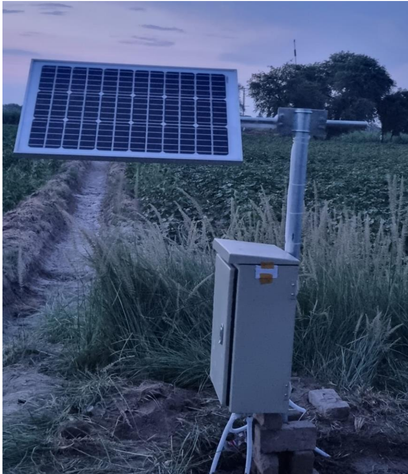
Site 9 – Diesel Pump – Rahim Yar Khan
