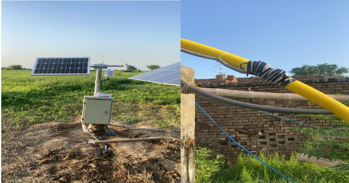
Site 4 - Solar Pump - Talagang
