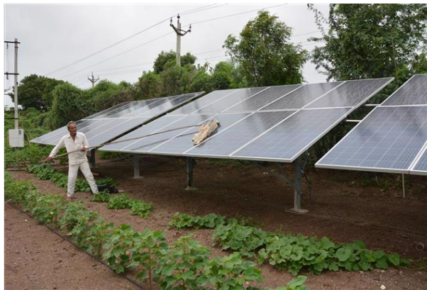
A farmer cleaning solar panels at Parmeshwar Feeder, Botad, Gujarat. Photo: Yashodha Yashodha/IWMI
