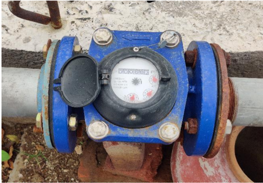
An installed flow meter. Photo: Md Faiz Alam/IWMI
