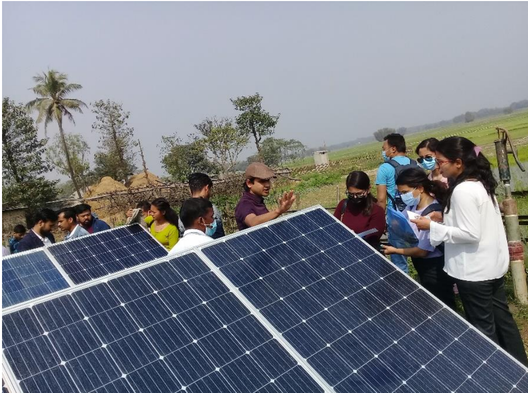
Figure 5: A site visit to Solar Irrigation Pump installation site in Jahada RM
