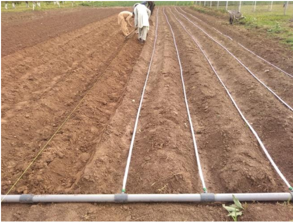
Picture 2: Trenching and RDI installation
